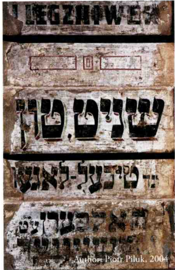
A Yiddish inscription (1) preserved on the wall of a building in Naliwajka St.
