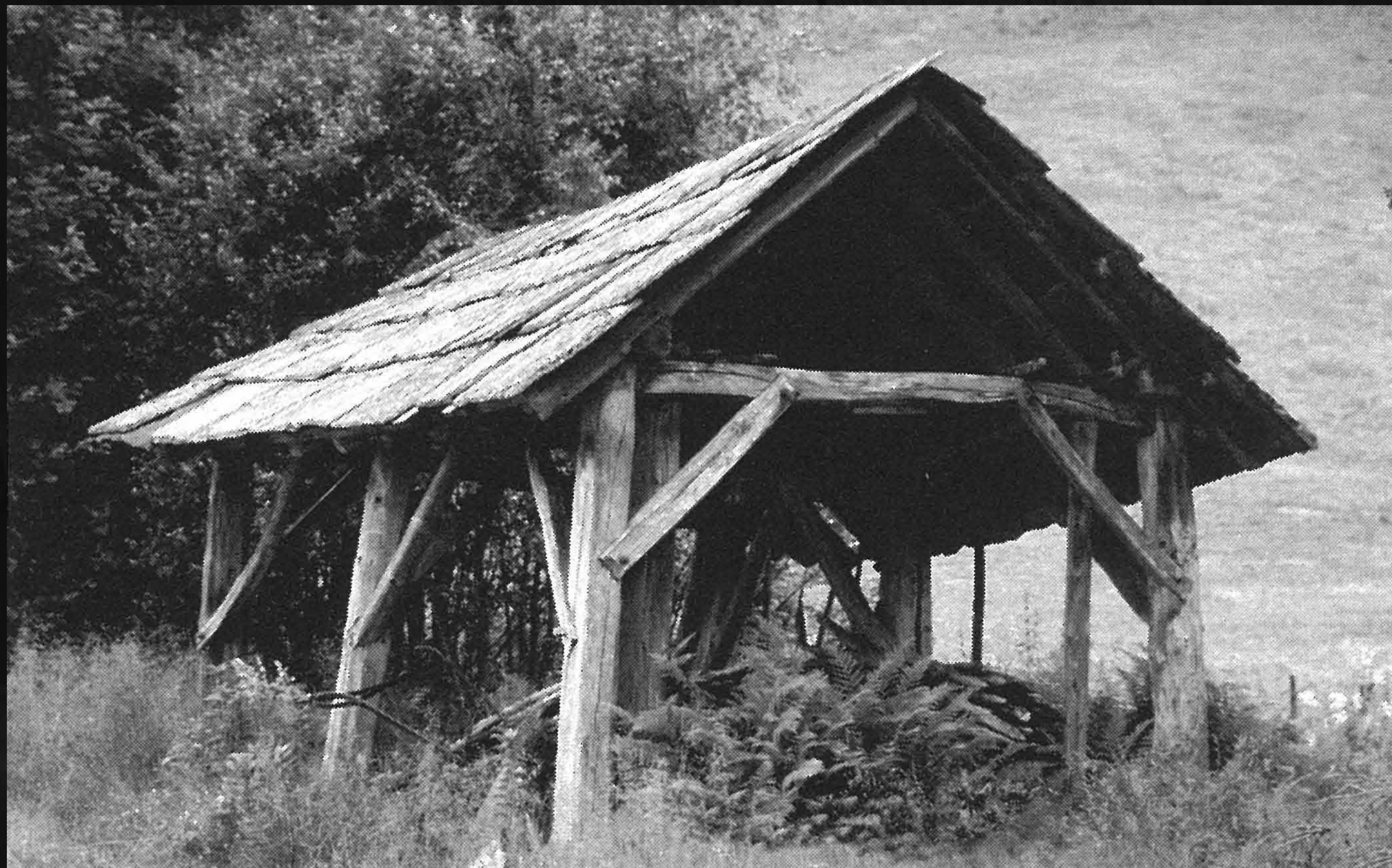
Trestle frame building from Øystese municipality Hordaland county. Photo by Helge Schjelderup
