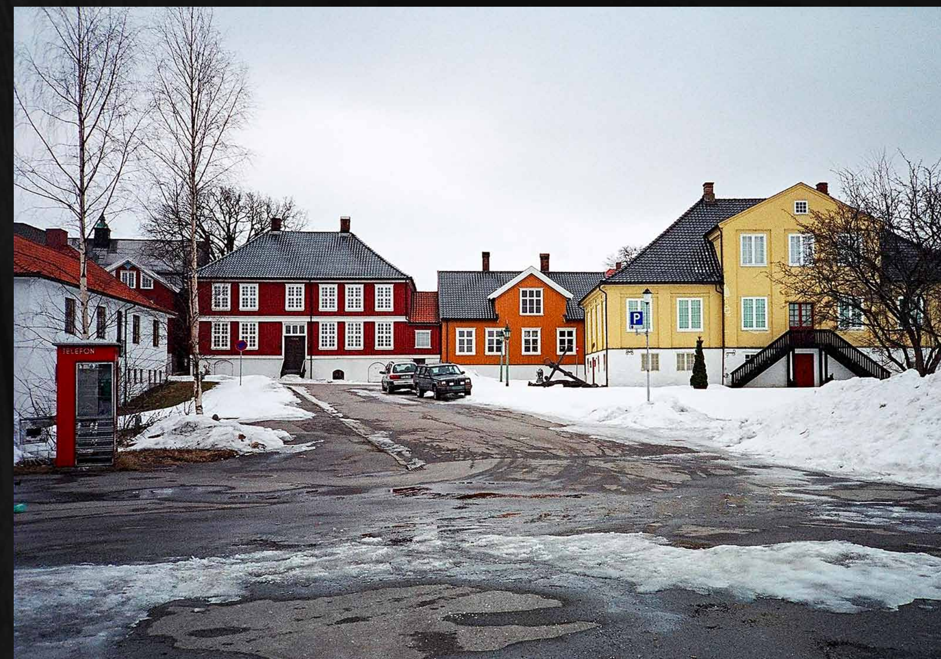
Houses in the former main street Storgata (now Kirkestredet), built by wealthy merchants and county officials in the first half of the 18th century. Photo by Lars Jacob Hvinden-Haug 2004
