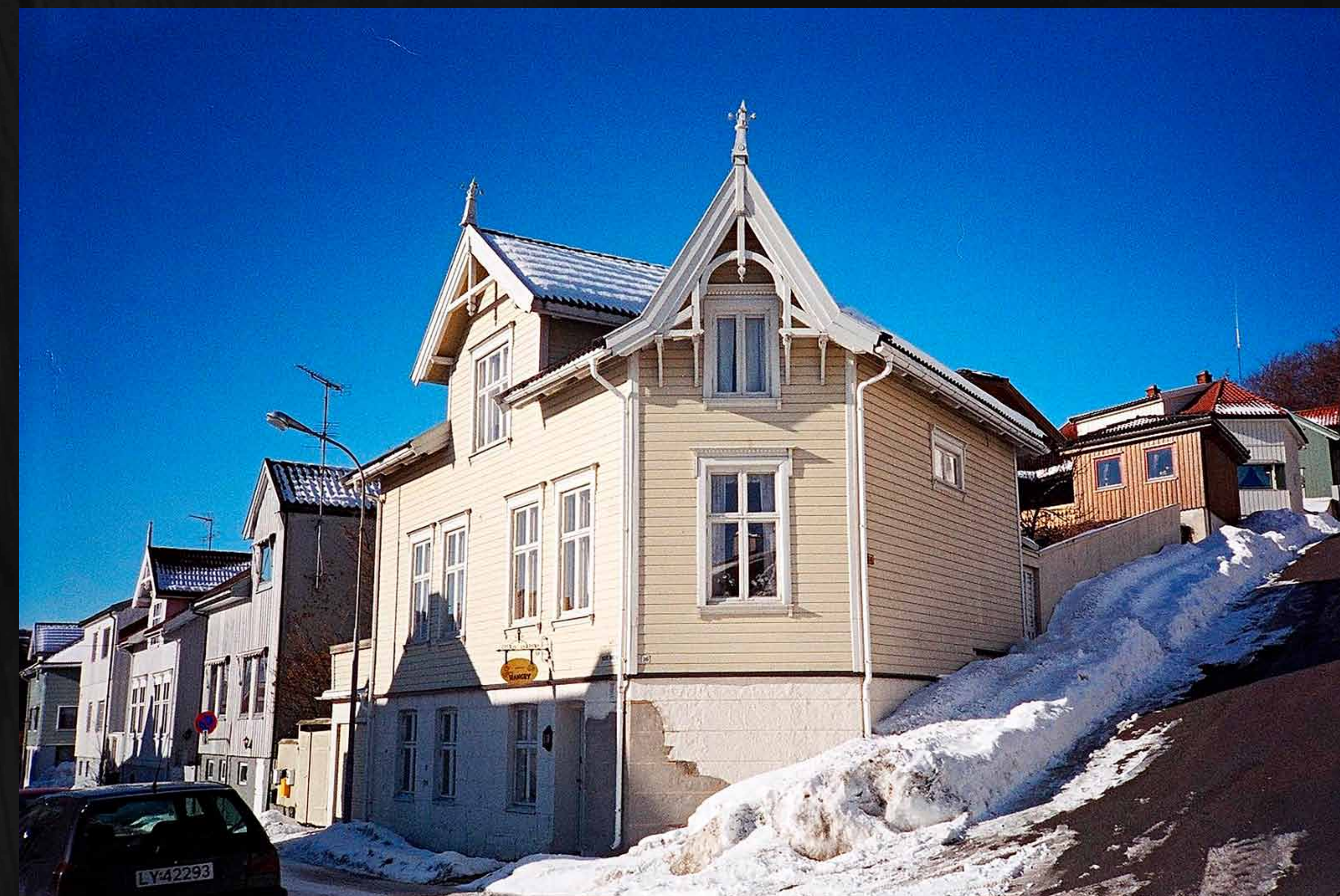
Nedre Bøkeligete 16. Typical dwellings of craftsmen and petty bourgeoisie in Steinane – late 18th Century. Photo by Lars Jacob Hvinden-Haug, 2004
